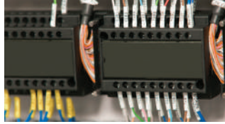
Cable wrap for electrical marking
